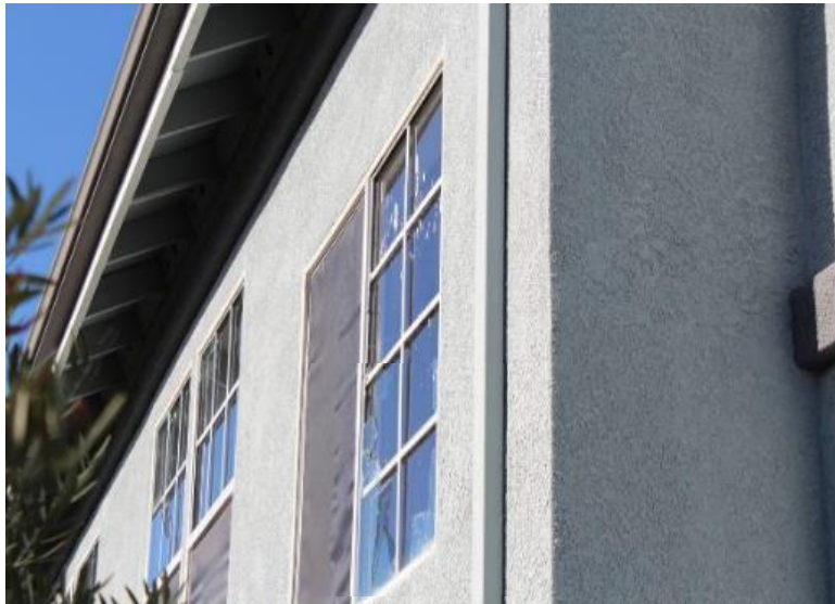
Double-Paned Window – Mitigation against flames & embers
